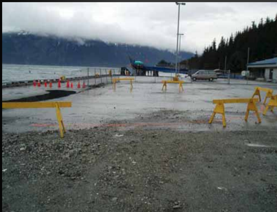
Sink holes and loss of fill
