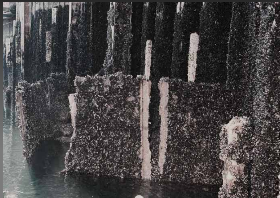
Corrosion failure closure arc (PND Engineers)
