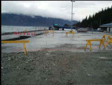
Sink holes and loss of fill
