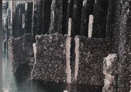
Corrosion failure closure arc (PND Engineers)
